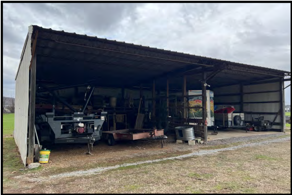
Photo 4: View of shed near the central portion of the Subject Property.
